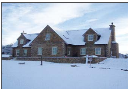
Airtight and energy efficient with consistent internal air temperatures
