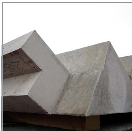
Bespoke connection detail created during manufacture to assure accuracy and strength
