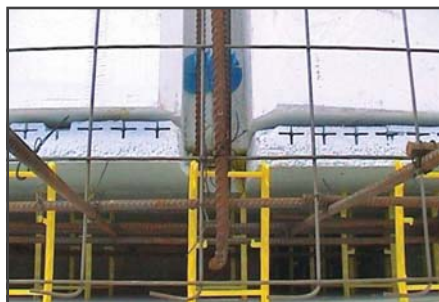
Horizontal and vertical structures are stitched with right angled rebar
