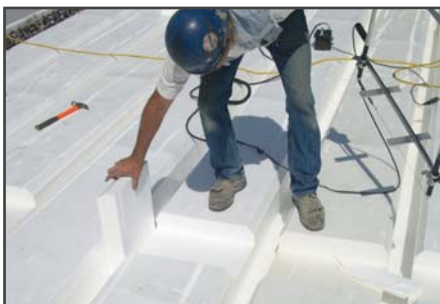
Slots are removed for cross beams
