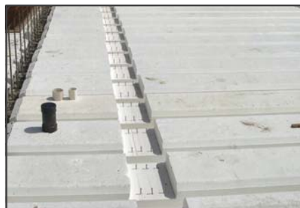
Drain and service pipe work can be easily placed through the panels
