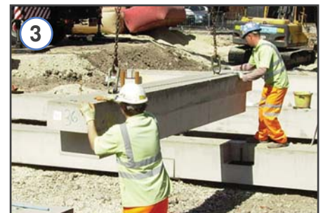
Rapid offloading and placing into position
